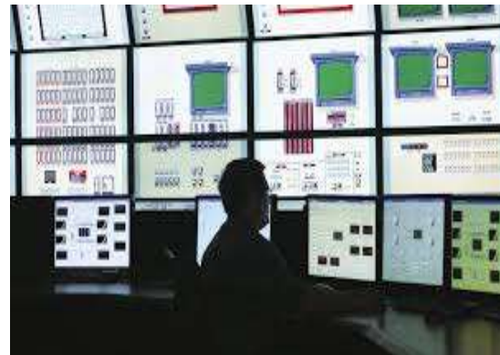
Critical Energy Infrastructure
